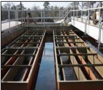
Fig 1: A typical coagulation tank in a drinking water treatment facility.
